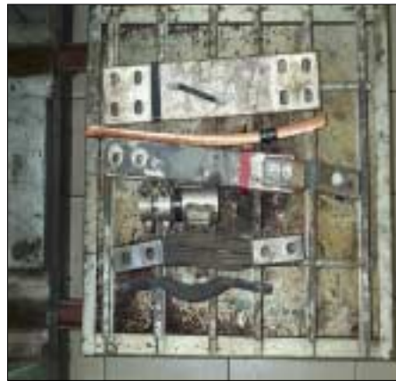
Figure 7. Electrical components taken out from the oven at 80^{\circ}\text{C}
